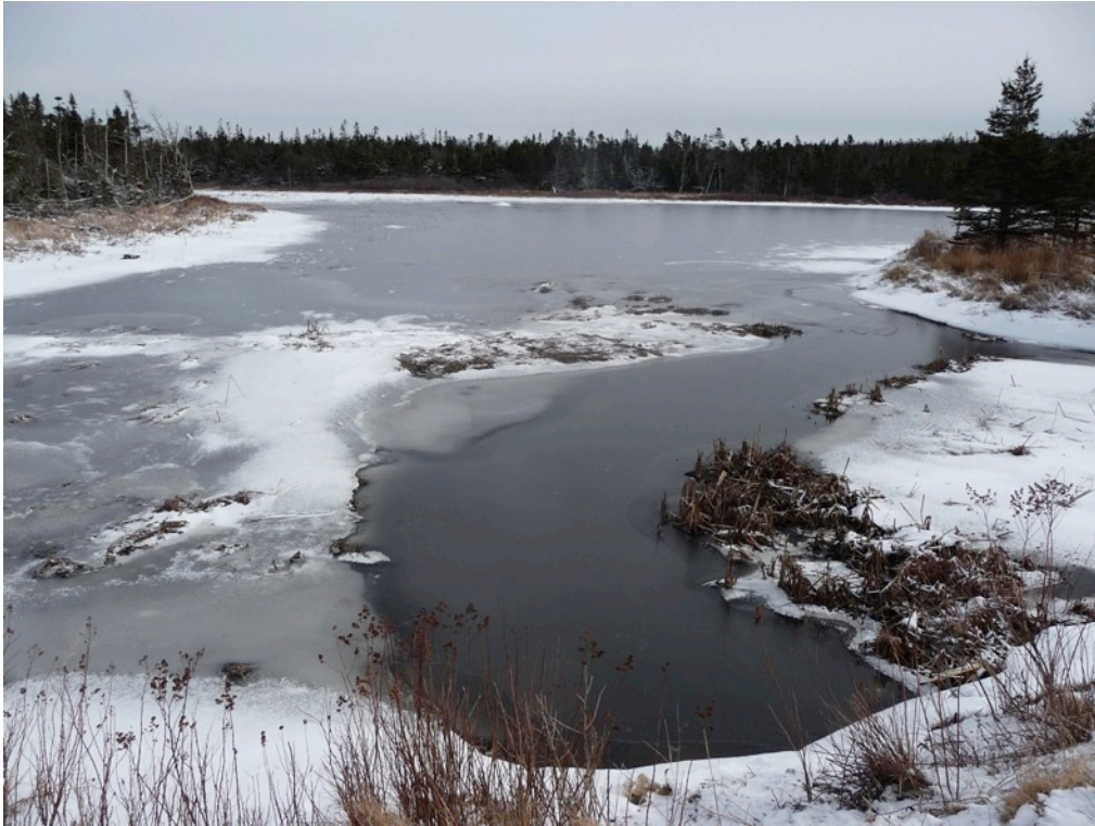
Figure 4 Upstream side of culvert and road.
