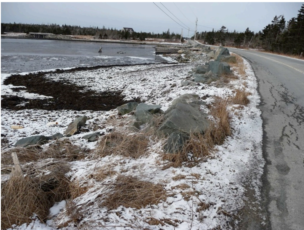
Figure 5 Downstream side of culvert and Three Fathom Harbour.
